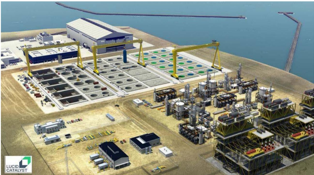
Figure A1.1 – Conceptual illustration with modular manufacturing and assembly building at rear, hydrogen gigafactory under construction beneath the yellow cranes, adjacent hydrogen manufacturing plant and liquid synthetic fuel manufacturing plant in the foreground
